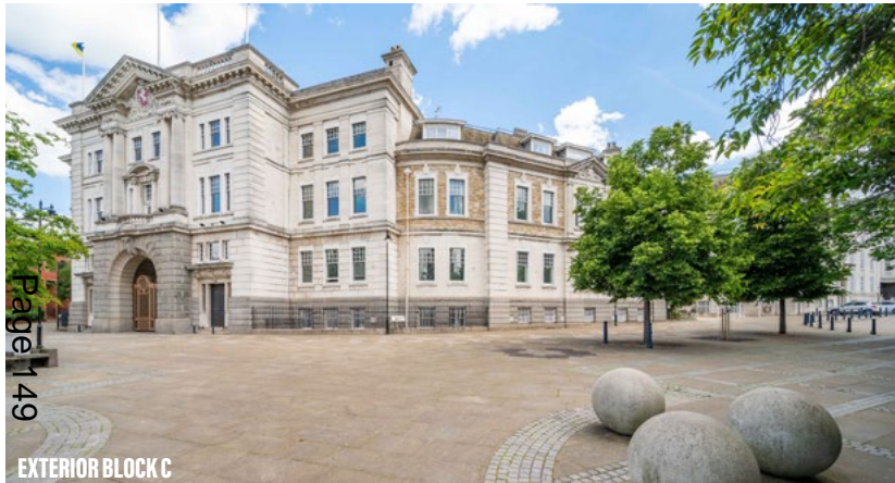
EXTERIOR BLOCK C
